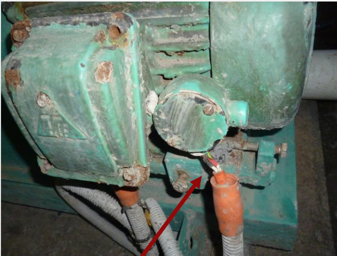
Exposed cables – terminals – potential “live”
